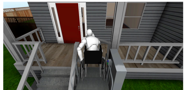
Figure 2: Entrance modified with a vertical lift
