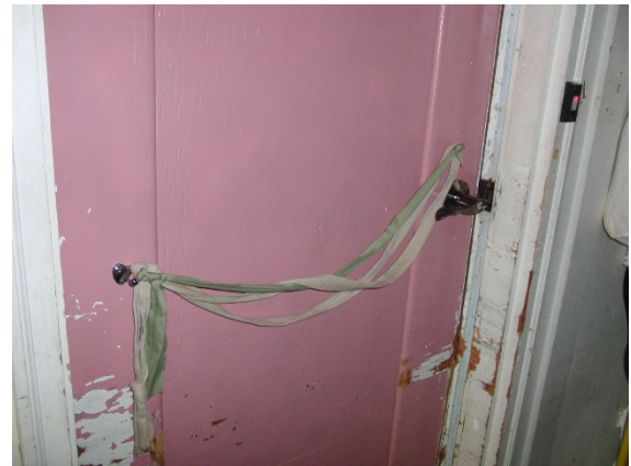
Figure 1. Example of a homemade door pull. Damage from the user's wheelchair to the doorframe can also be seen.
