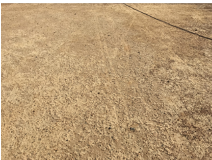
Figure 3. Packed dirt testing
