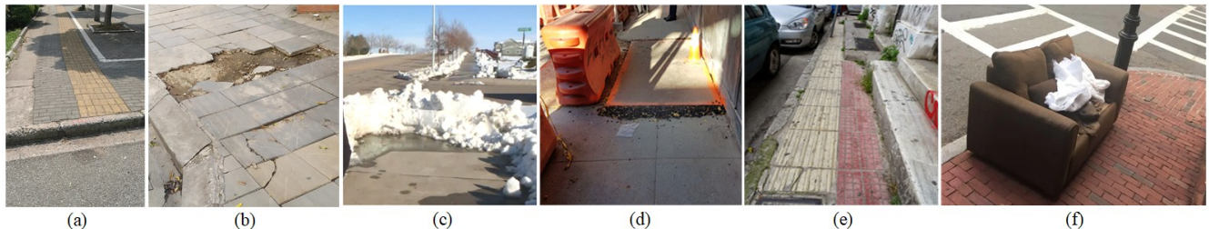
Figure 1. Barriers found in the built environment: (a) Curb with no access ramp, China, (b) Broken sidewalk, Vietnam, (c) Snow piled on sidewalk, Omaha, USA, (d) Construction, NYC, USA, (e) Narrow sidewalk, Athens, Greece, (f) Discarded furniture, Boston, USA
